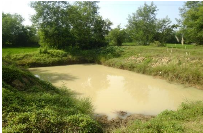
Fig. 4 Mud excavated rain water harvesting structure known as Happa
